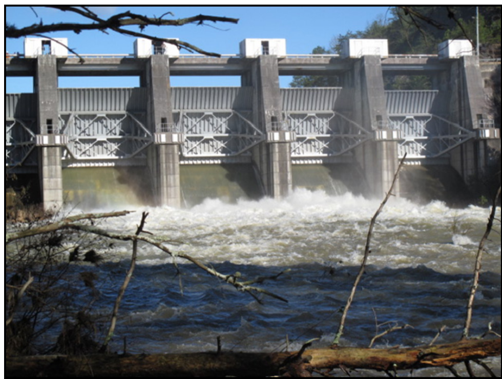
Figure 2-11 Upstream View, Emergency Spillway Releasing Approximately 4,000 cfs
