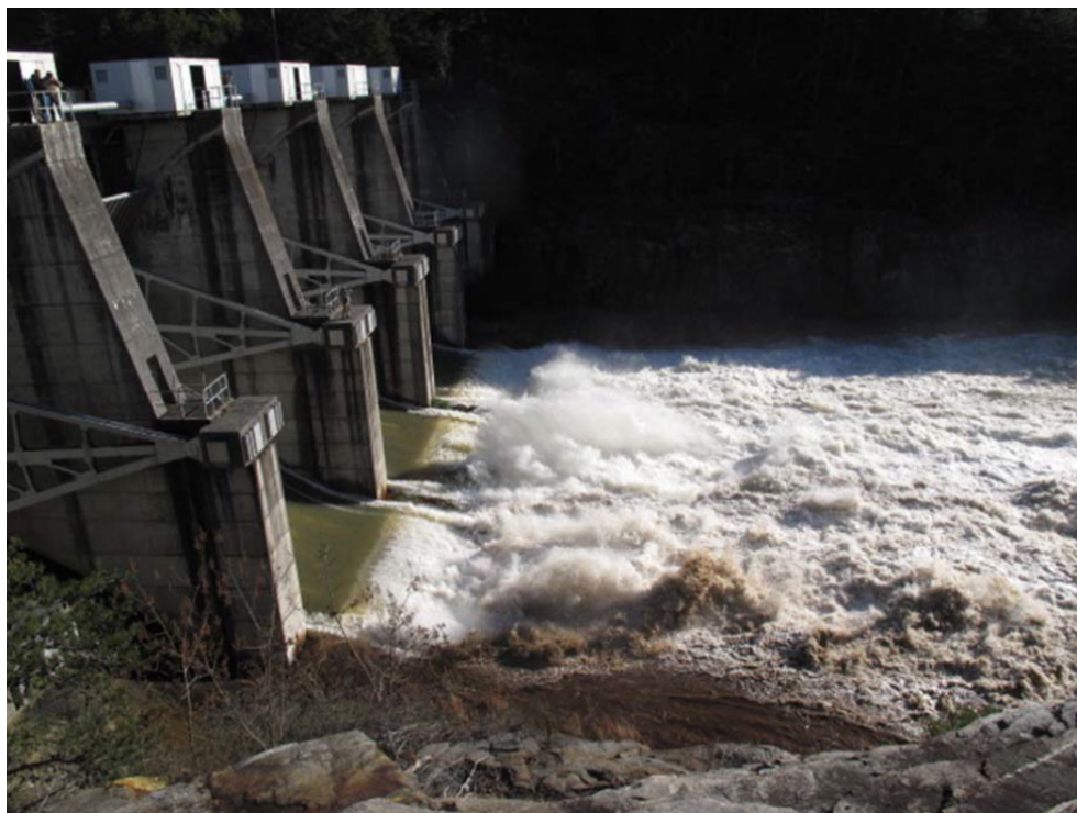
Figure 2-10 East View, Emergency Spillway Releasing Approximately 4,000 cfs
