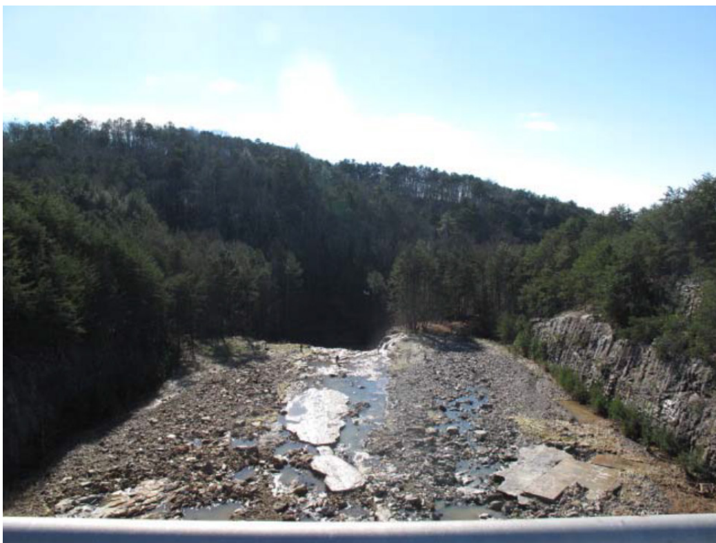
Figure 2-15 Downstream View, Emergency Spillway Channel After Test
