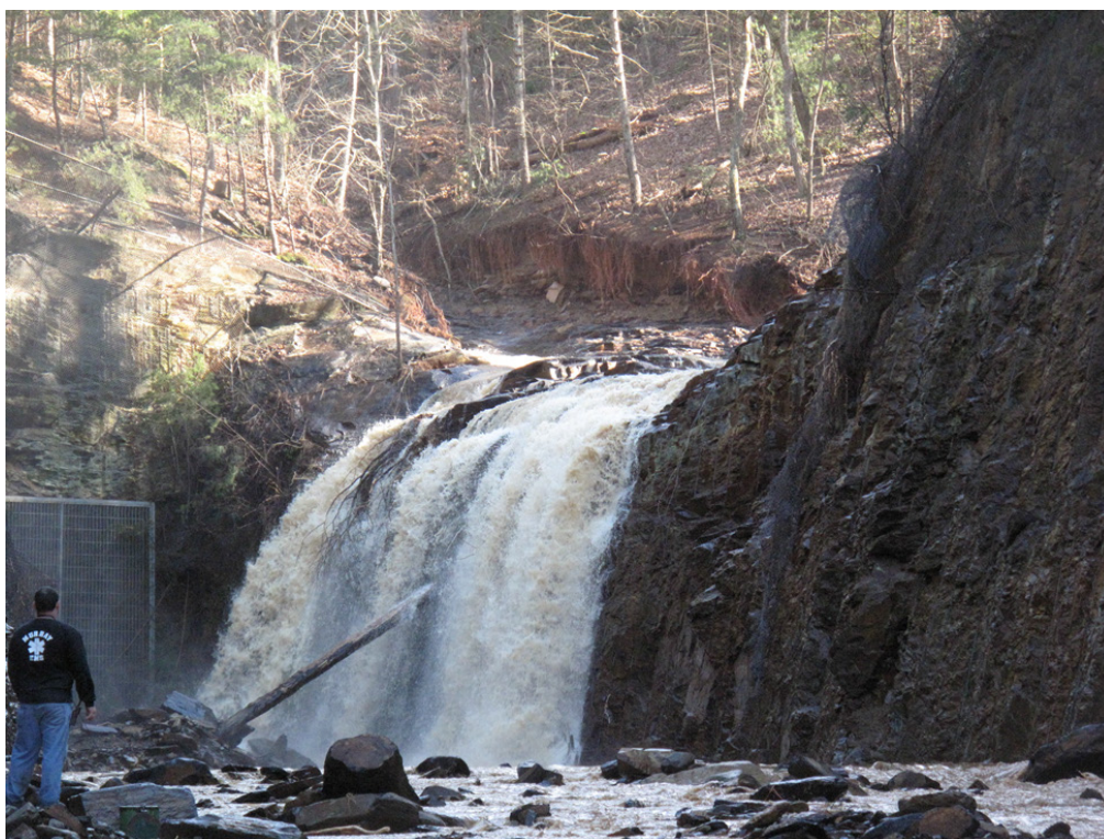
Figure 2-13 Emergency Spillway Channel Downstream Outlet, Adjacent to the Sluice Tunnel Outlet During Test Release
