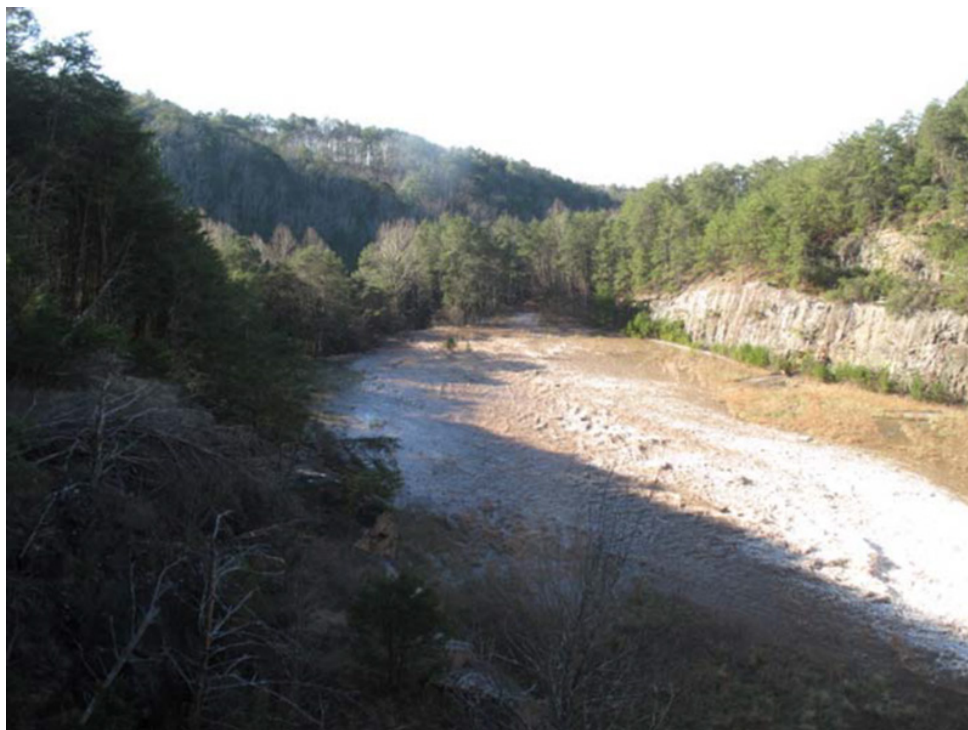
Figure 2-12 Downstream View, Emergency Spillway Releasing Approximately 4,000 cfs
