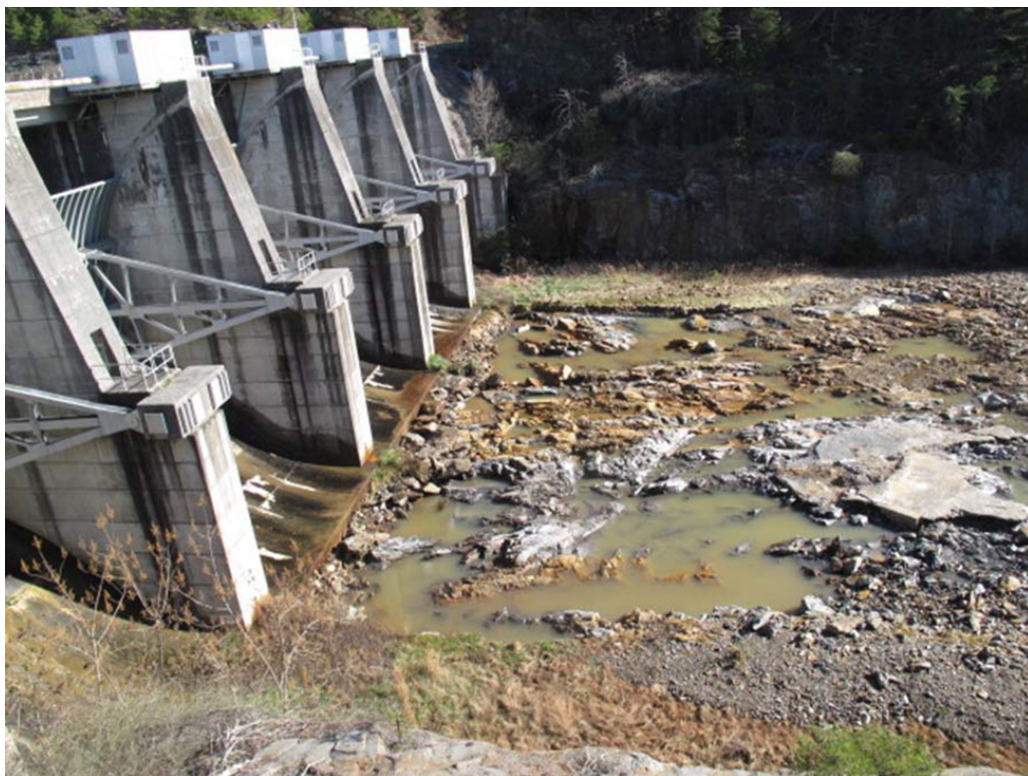
Figure 2-14 East View, Emergency Spillway and Channel After Test
