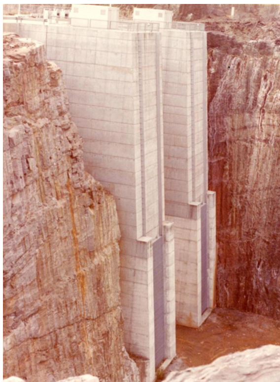
Figure 2-18 Right Bank Intake Prior to Filling, Circa 1974
